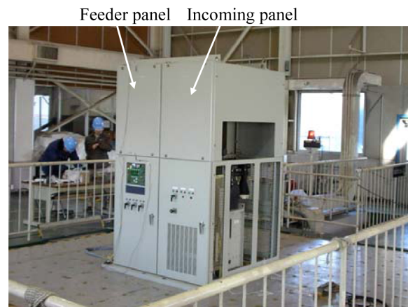
Fig. 8. Seismic test setup.
